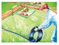
Unroll the polythene coil, from the valves to the stakes, along the marked path. Put the "I" or connector couplings and the drainage valves in the position for installation. Straighten the tube properly before cutting it to length (better too long than too short). Use a hacksaw to cut the tube; clean cut ends with a scraper before fitting compression connectors to ensure a completely watertight connection.
